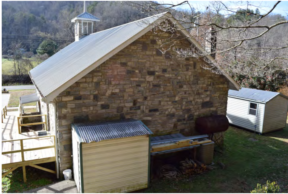
Rear elevation and two small storage buildings, view to the west
