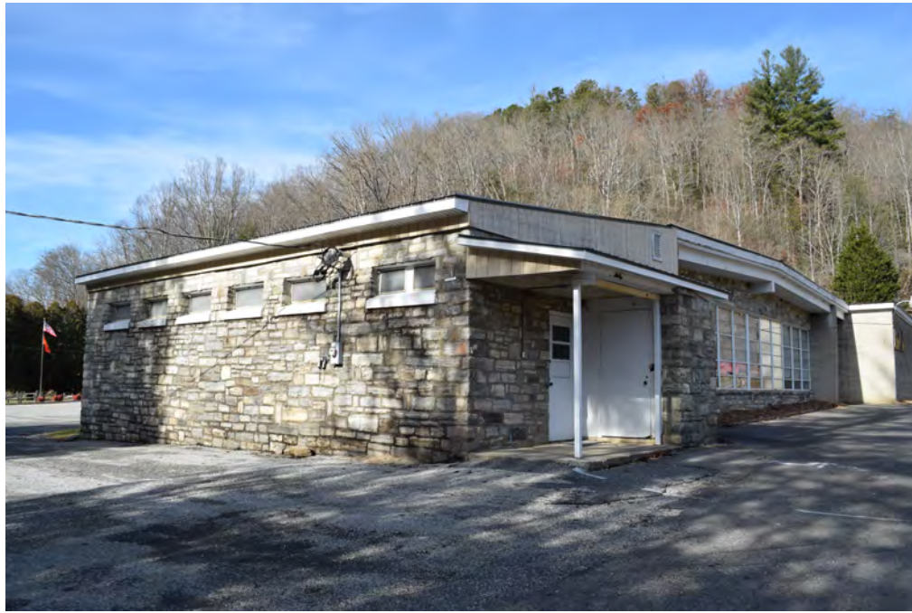
1958 Addition to Alarka School
