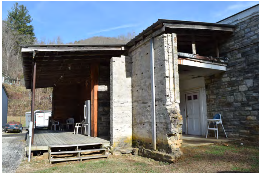
West elevation of 1958 addition, view to the north
