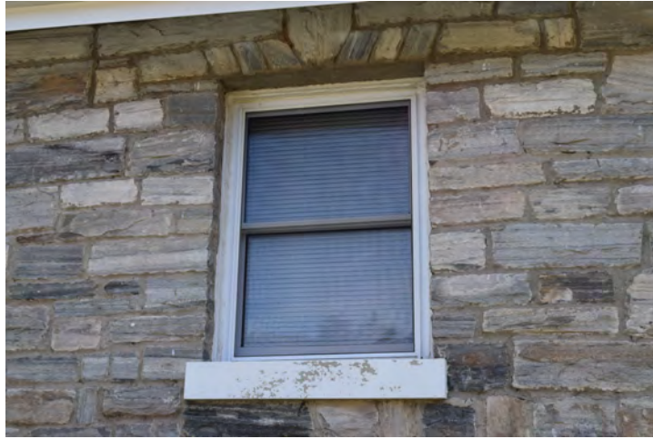
Detail of north elevation window, view to the south
