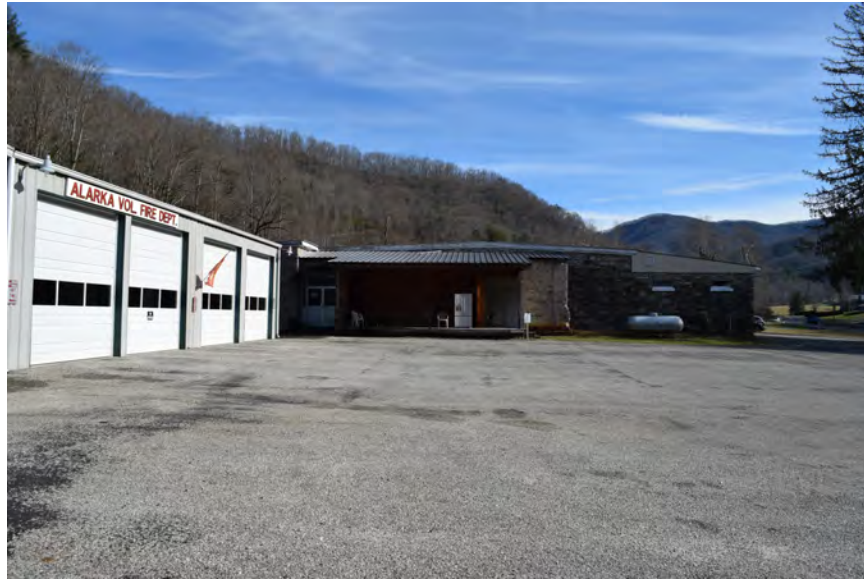
Modern fire station at the site of Alarka School and west elevation of 1958 addition, view to the east
