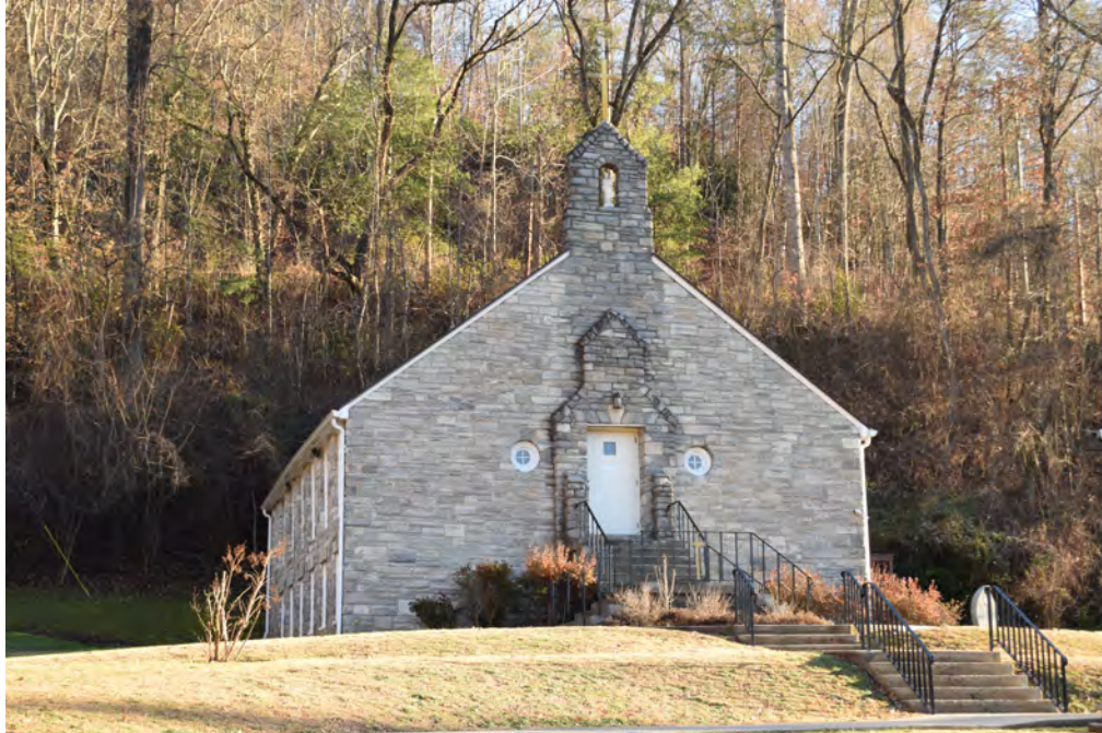
St. Joseph Catholic Church built in 1941 in Bryson City, view to the south
