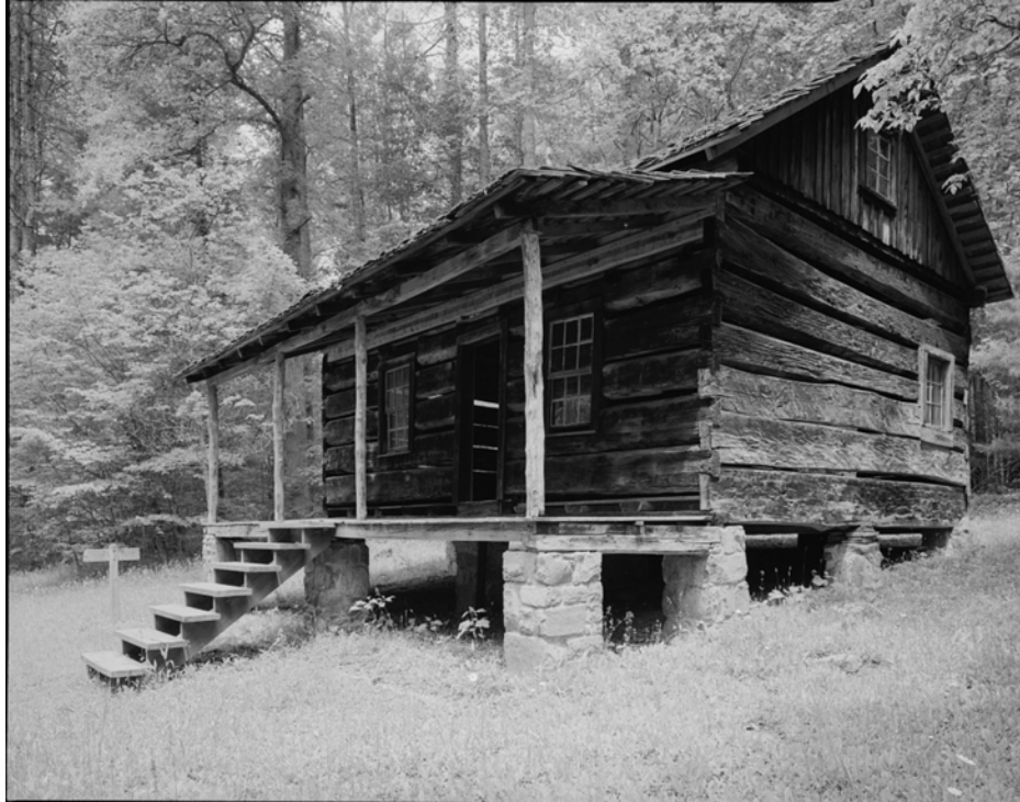
J. H. Kress Cabin, Historic American Building Survey (HABS) photo from Library of Congress website, view to the northeast
