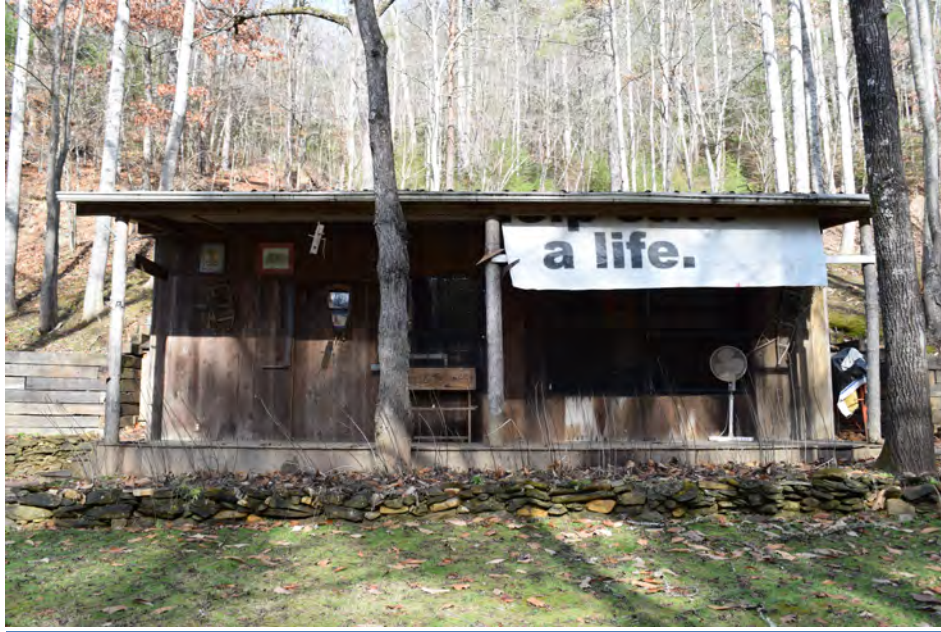
Shed located to the east of the Oliver-Gibson House, view to the north
