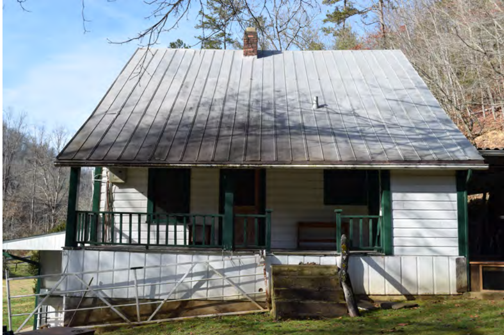
Oliver-Gibson House rear elevation, view to the northwest
