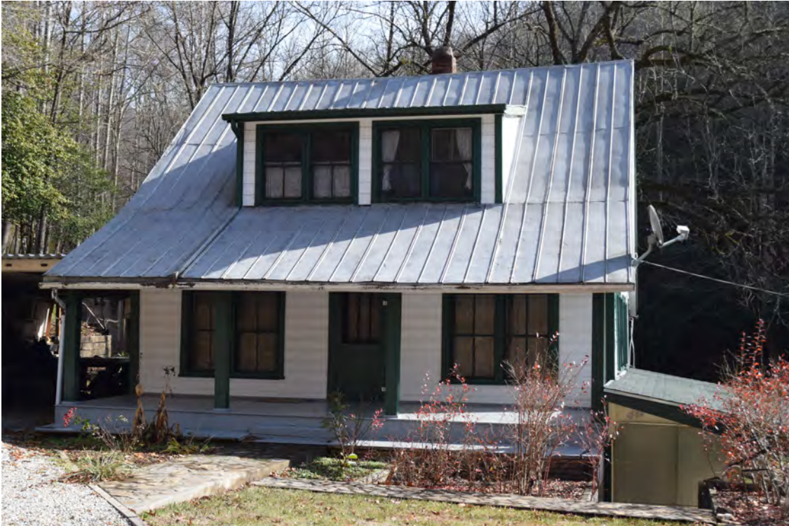
Facade (west) elevation of Oliver-Gibson House
