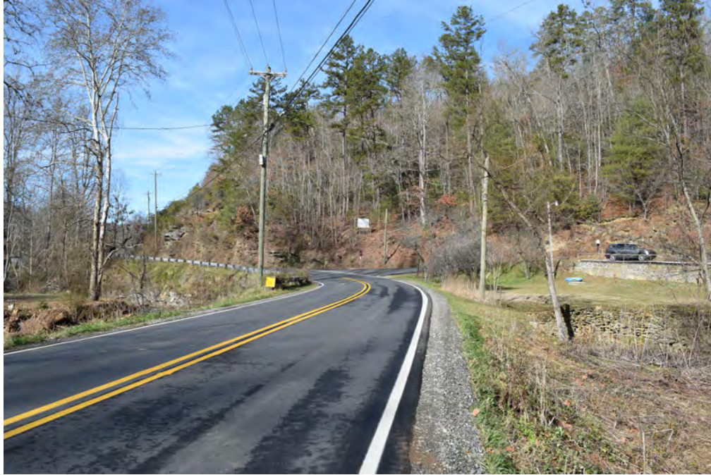
Alarka Road (SR 1140) with Little Alarka Creek to the right and Alarka Creek to the left, view to the north
