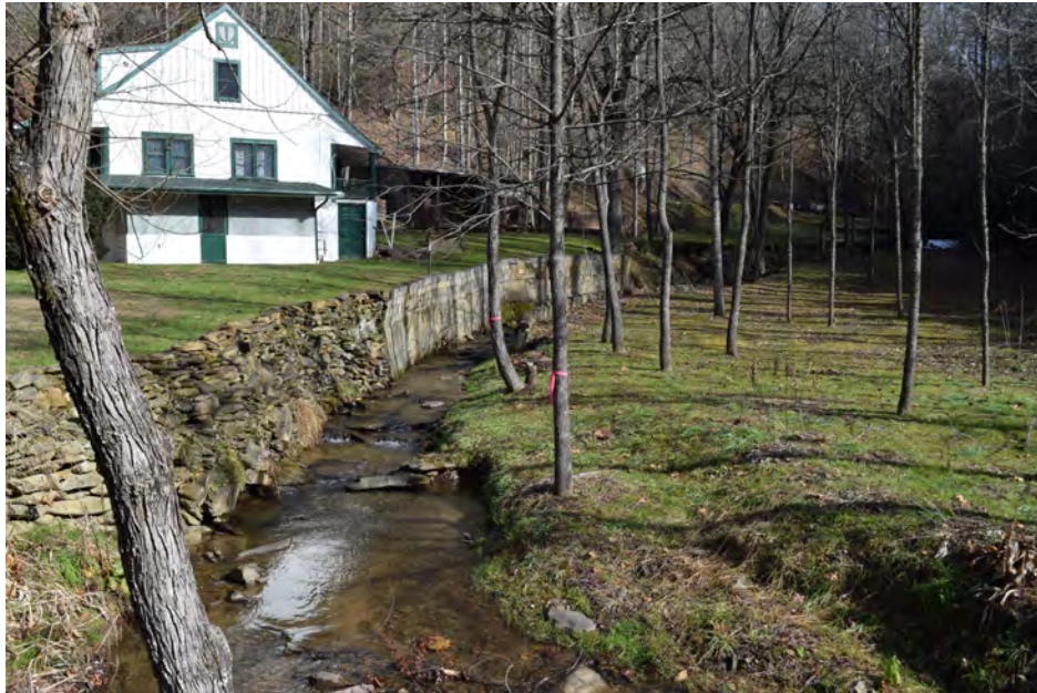
Oliver-Gibson House, west elevation, and Little Alarka Creek, view to the east
