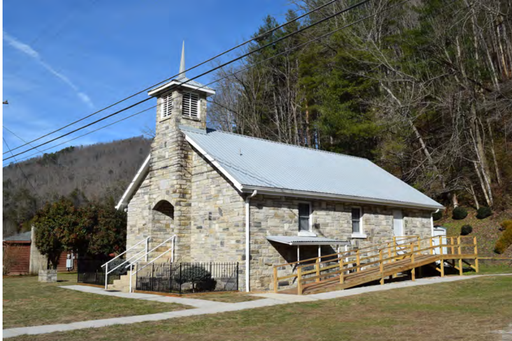
Southwest corner of the church, view to the north-northeast
