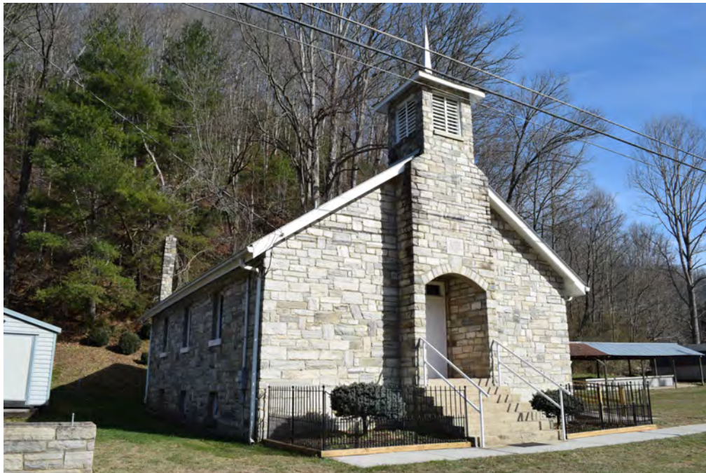
Northwest corner of church, modern storage building, view to the southeast
